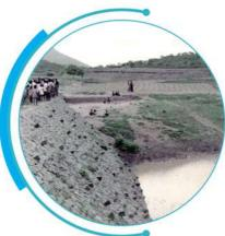
From 1979 to 2002, IVDP implemeted watershed programs around the hills of Anjetty Region. This involved with planning and construction of 92 major and 239 minor check dams, built across streams and gullies in the hilly region. The check dams are designed to retain monsoon rains, leading to the increased groundwater levels and storing water for the irrigation, livestock and domestic requirements of the villagers.
